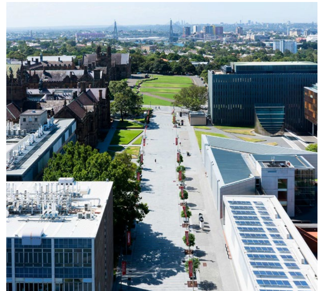
Above: Drone footage of Eastern Avenue solar panels on Camperdown Campus, part of our effort to generate 3 megawatts of on-site renewable electricity by 2025. Previous page: Organics Waste Trailer in front of the Michael Spence Building on Camperdown Campus, awaiting activation of "Chester the Biodigester"
