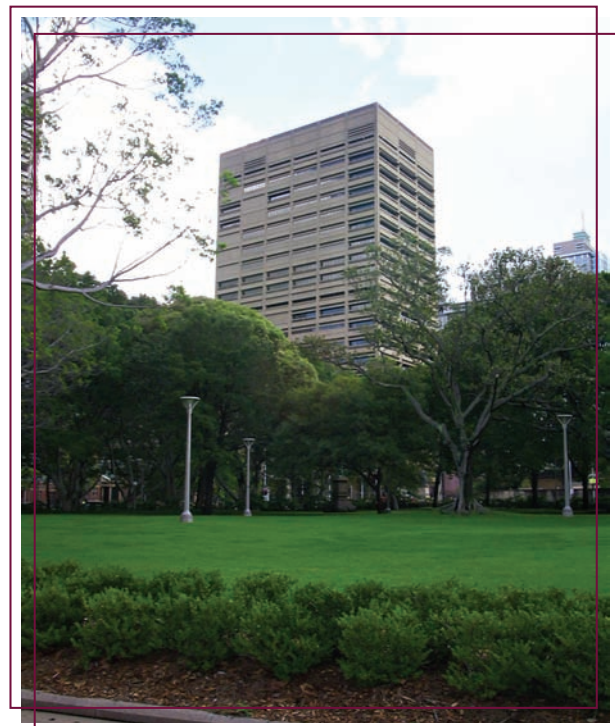
NSW Law Courts Building
