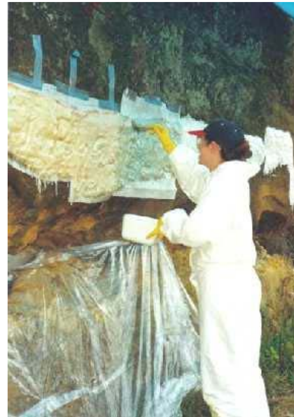
Felicity Quinlin applying the fibreglass jacket
